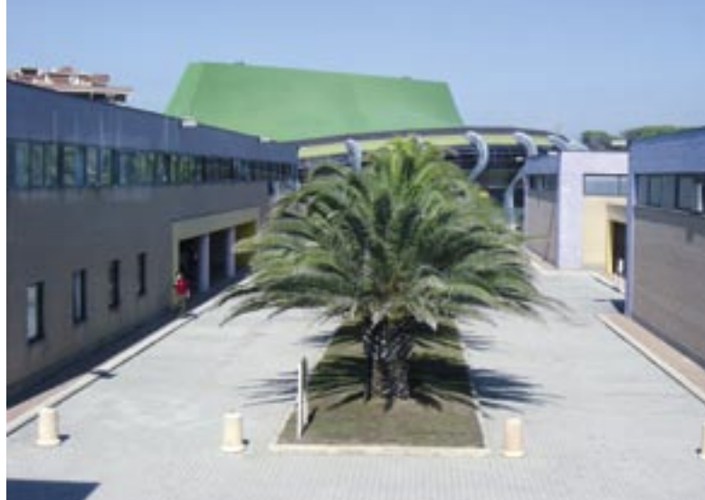
I servizi The facilities
