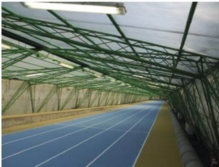
La pista coperta The indoor track
